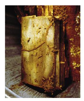
Figure 16. Warm, moist wood provides subterranean termites with all of their survival requirements. (B.T. Forschler)
