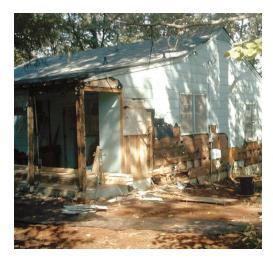
Figure 17. The siding was removed from the porch and an exterior wall of this house to show the extent of termite damage. (B.T. Forschler)
